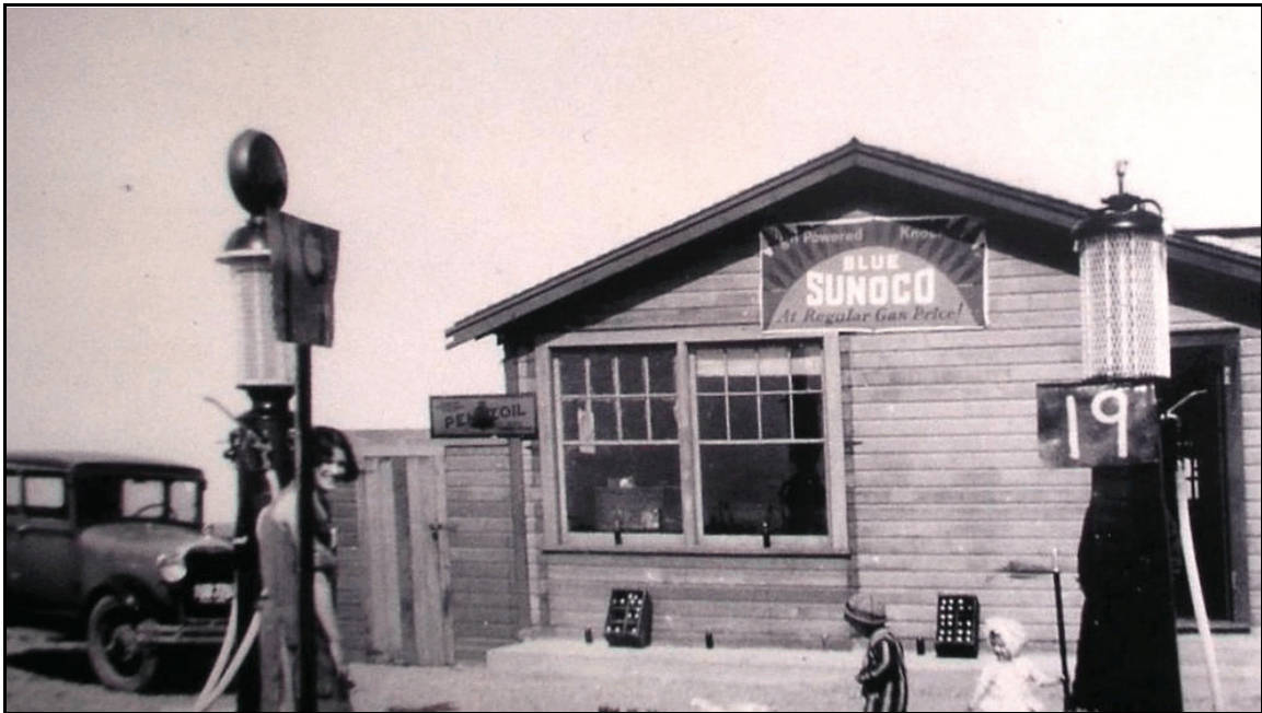
A curbside pump located at North Federal Heights Grocery & Supply Station, 93 rd & Federal. Owned by Harvey Larsen. Photo courtesy of the Westminster Historical Society.
