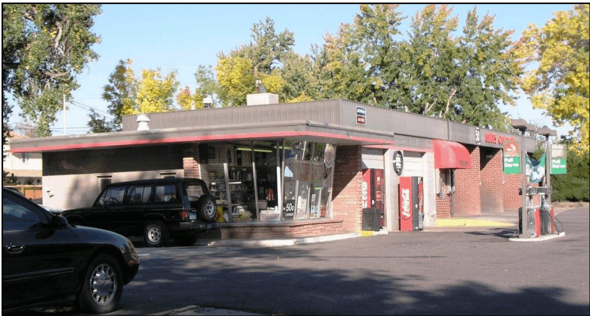
Herb's Service Station at 3791 W. 72 nd Avenue features flagstone veneer and angled display windows in the office area. The car wash bays on the right are a later addition.
