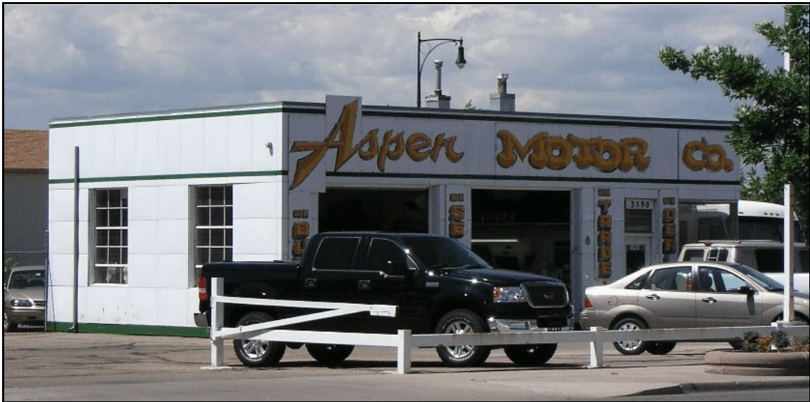
An oblong box with porcelain steel siding and angled corner at 3590 W. 72 nd Avenue.
