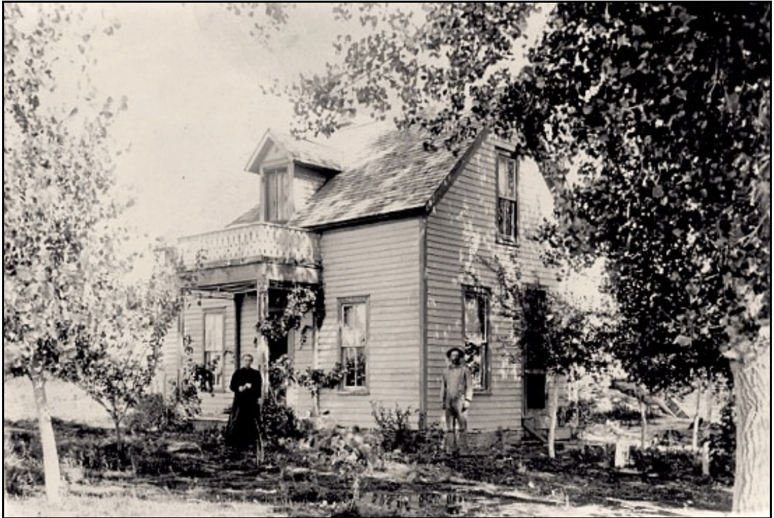
Pleasant and Sarah DeSpain's house on W. 76 th Avenue (demolished). Photo courtesy Westminster Historical Society, date unknown.
